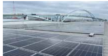
IIF Osaka Suminoe Logistics Center I
