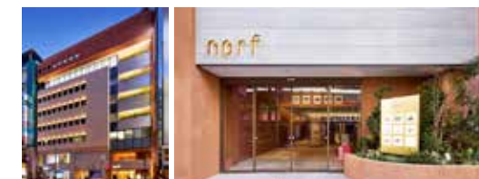
Renovated exterior 1F entrance hall
