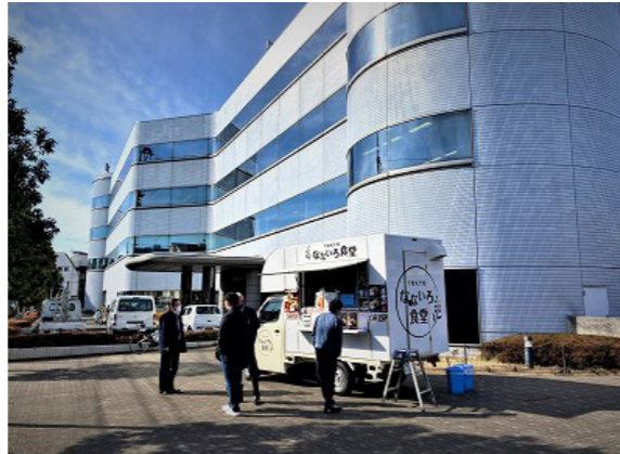
IIF Shinagawa Data Center
