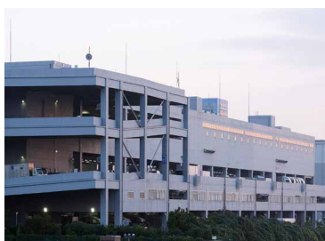
IIF Shinonome Logistics Center
