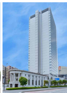
Yokohama i-land Tower
