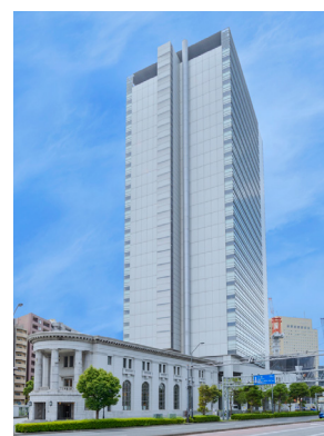
Yokohama I-land Tower
